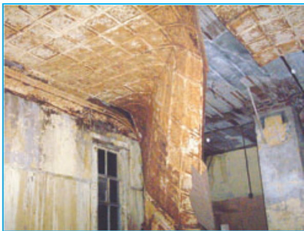
Deteriorated ceiling.
